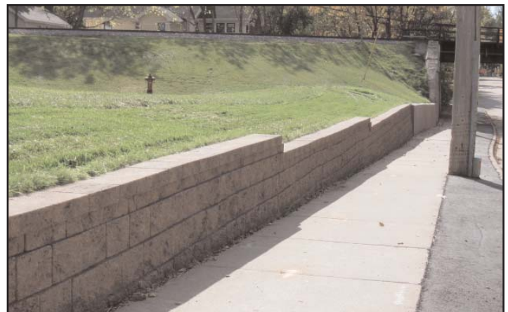
Mason Street Retaining Wall
